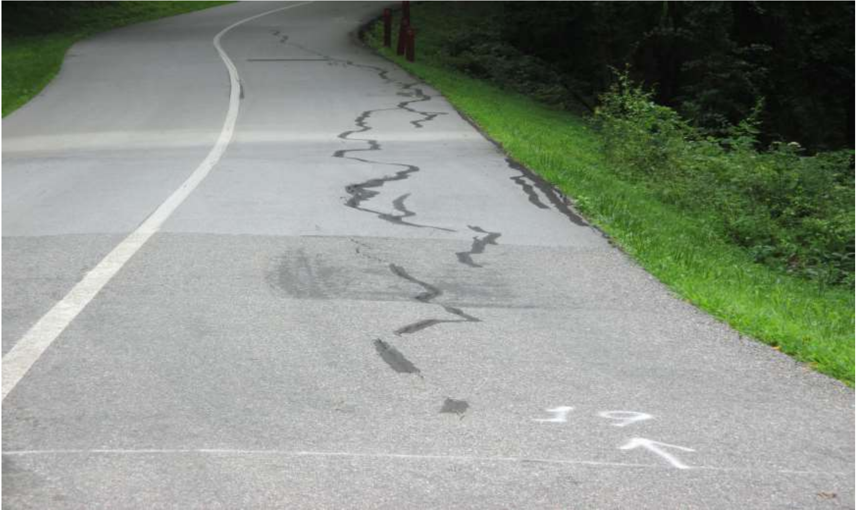
High Vista Drive at the Honey Locust stop sign, Cracks filled 8 months ago
