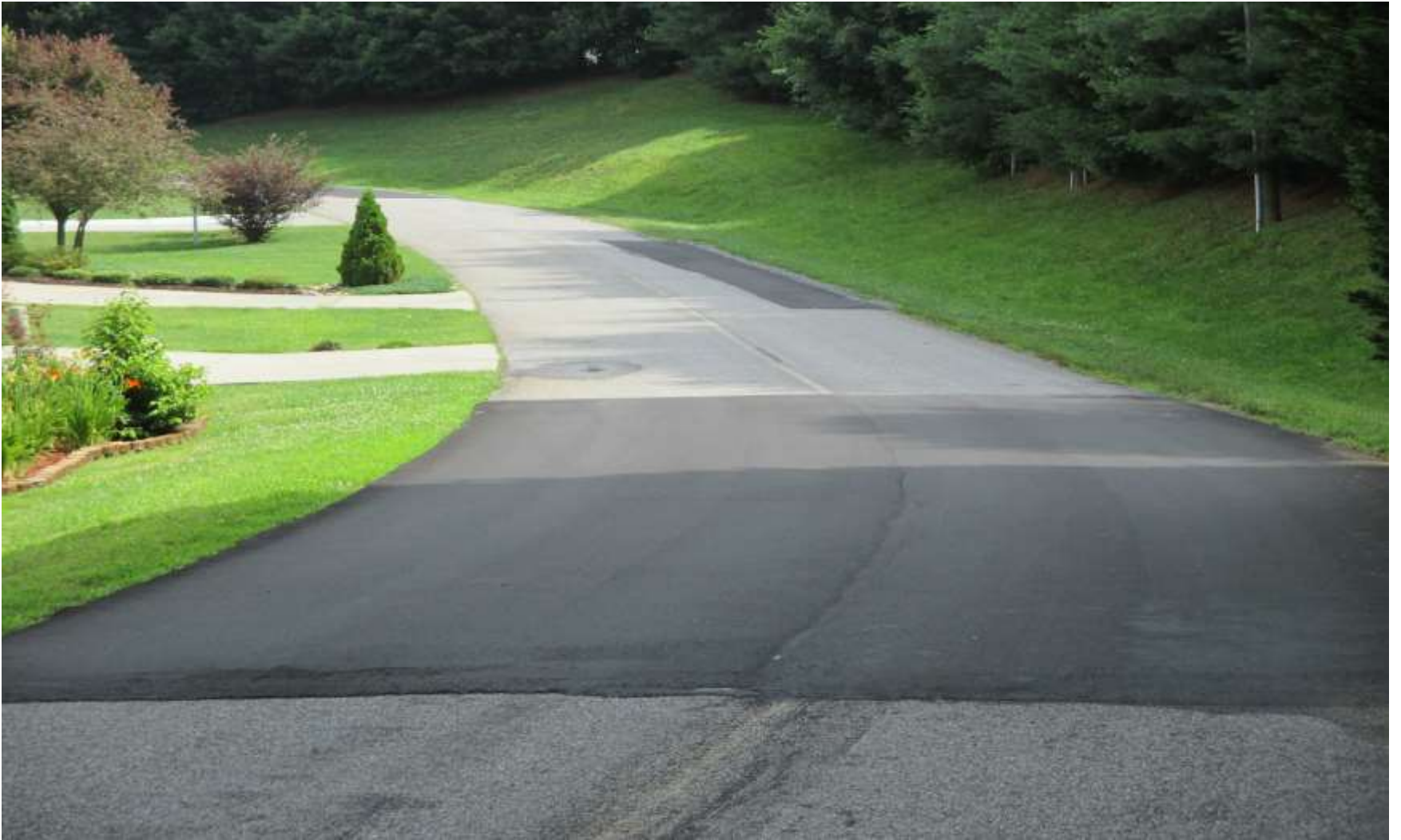
Vista Falls overlays completed last year
